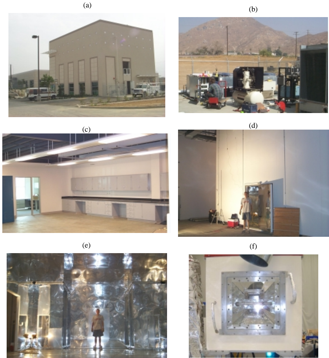
Figure 2. Selected photographs of the new environmental chamber building, enclosure and light source taken during its construction. (a) Outside view of laboratory building. (b) Construction of air purification and chamber refrigeration systems. (c) Laboratory room underneath new chamber. (d) Outside chamber enclosure in the upstairs laboratory. (e) Inside chamber enclosure looking towards the where the lights will be located, showing reflective materials on all surfaces, the access door, and the intakes for air handler. The light will be located about three feet directly above the person's head. (f) Argon arc lamp and enclosure (taken at the factory during its construction).
