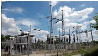
Substation: 69 kV / 12 kV
