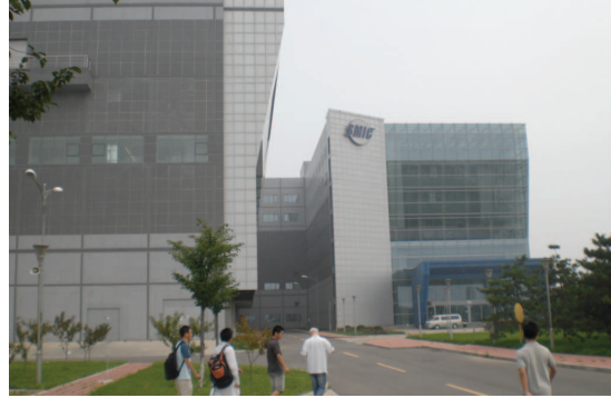
Figure B.12 On our way into SMIC foundry
