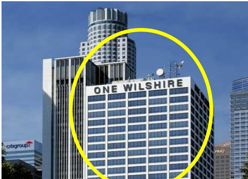
CoreSite's "One Wilshire" (Photo: CoreSite)
