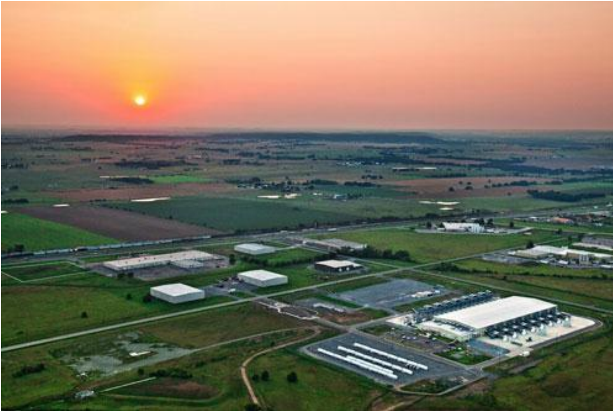
Google's data center in Mayes County, Oklahoma
