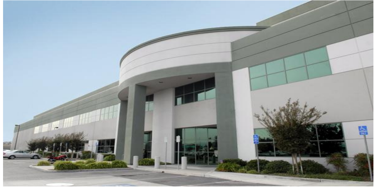
A data center in Santa Clara, CA
