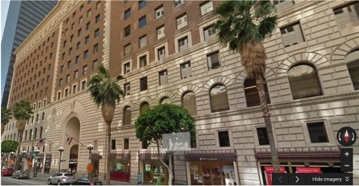
A "data center" located in 818 W. 7th Street, Los Angeles, CA 90017
